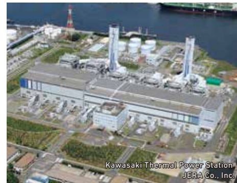
Gas Turbine Combined Cycle (GTCC) Power Plant
