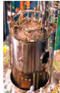
Replacement of Integrated Reactor Internals
