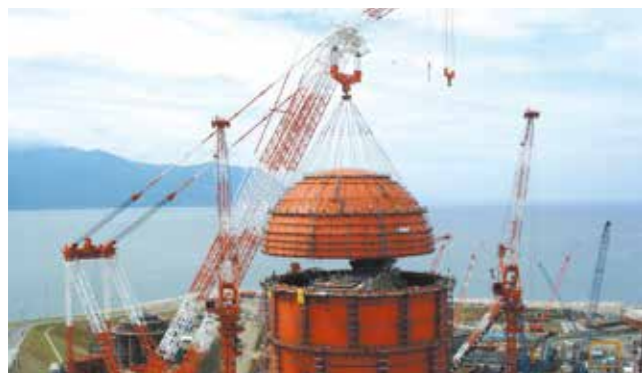
Construction at Hokkaido Electric Power's Tomari Power Station Unit 3
