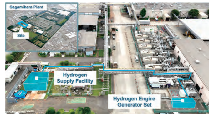
Figure 9 Installation site in Sagami-hara Plant (Starting in FY2024)
