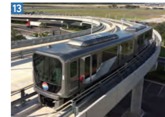
Tampa International Airport APM
