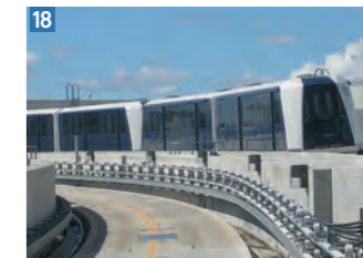
Miami International Airport North Terminal Skytrain APM
