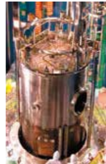
Replacement of Integrated Reactor Internals
