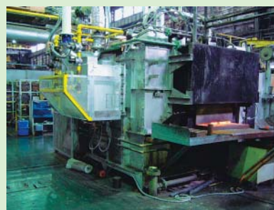
Waste heat recovery burner
