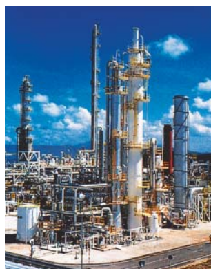
Urea production plant in Malaysia, where recovered CO 2 is effectively used as raw material for producing urea
