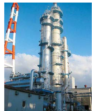
This CO 2 recovery plant in Fukuoka has the capacity to recover 283 tons of CO 2 per day.
