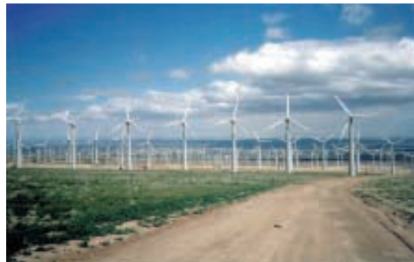
250 kW × 660 units/system Mojave Desert, California, U.S.A. The world's largest area (1.4 km × 1.1 km)
