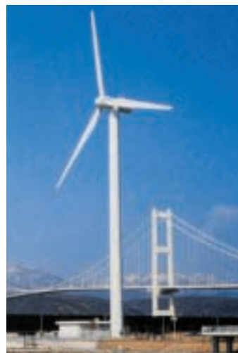
Muroran city, 1,000 kW system
