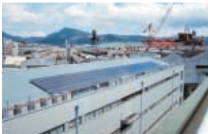
10kW field test system for factory use
