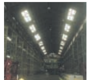
Natural light windows on factory roof
