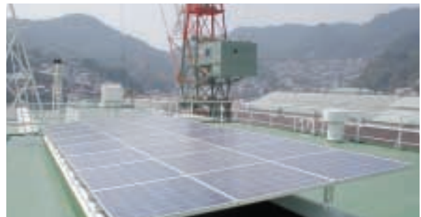
Solar Energy Generation System
