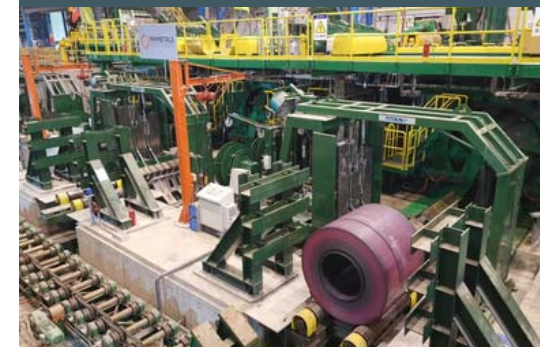
Rizhao Steel (China) launches its fifth ESP plant with equipment supplied by Primetals
