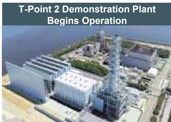
T-Point 2 Demonstration Plant Begins Operation Facility for long-term validation of next-generation high-efficiency JAC* class GTs, which were the first in the world to achieve inlet temperatures of 1,650°C *JAC: J-series Air-Cooled
