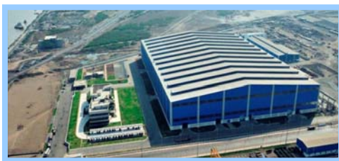
L&T-MHI Turbine Generators
