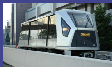
APM at Singapore Changi International Airport
