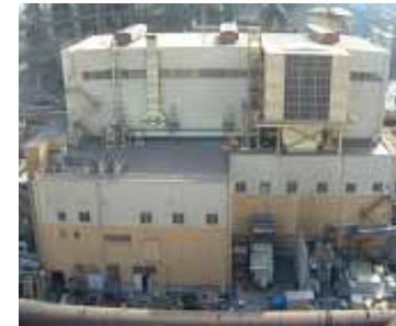
World's largest BFG-fired GTCC (using M701F)
