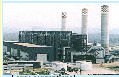
Large conventional power plant
