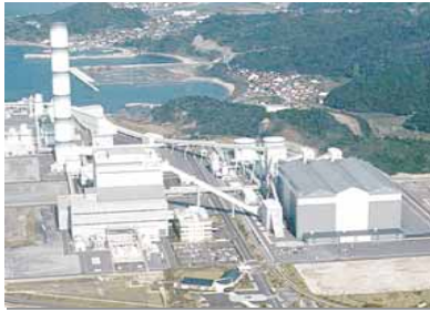
Ultra – Supercritical Pressure Power Plant
