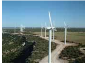
Wind Power Generation
