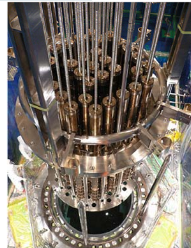
Core structure replacement
