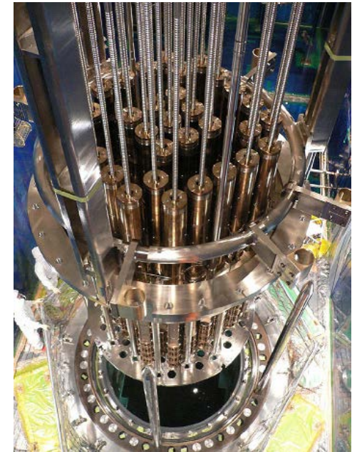
Core structure replacement
