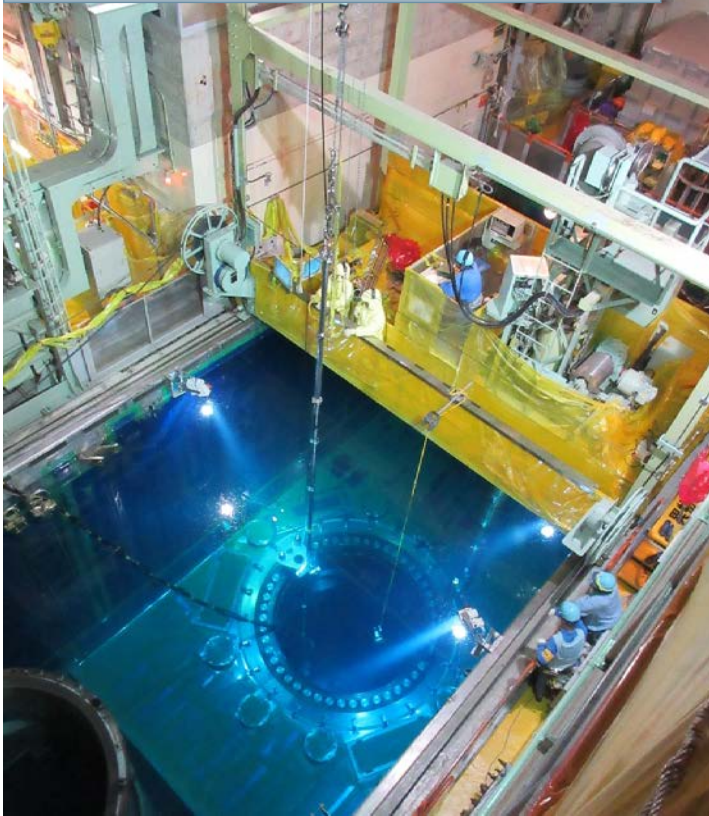
Light water reactor decommissioning Sampling inside reactor vessel
