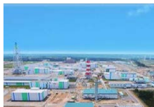
Rokkasho Reprocessing Facility
