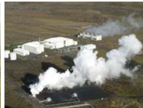
Iceland Nesjavellir Power Plant
