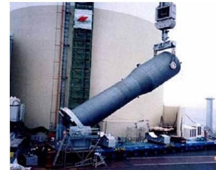
Steam generator replacement work
