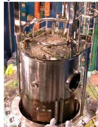
Reactor internal replacement work
