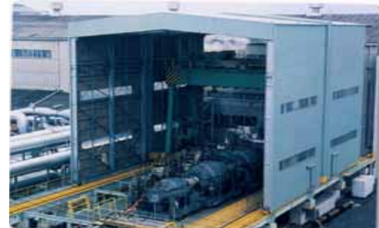
* E.g. Installing extra large testing facilities
