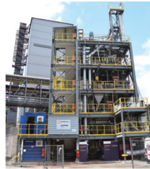
The HYFOR pilot plant in Leoben, Austria
