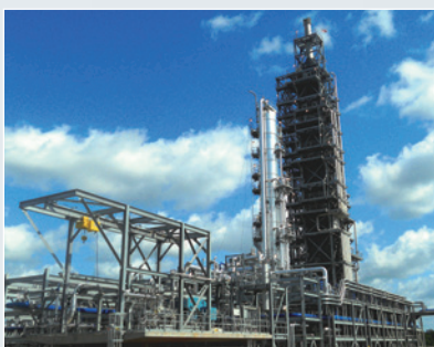
CO 2 capture plant
