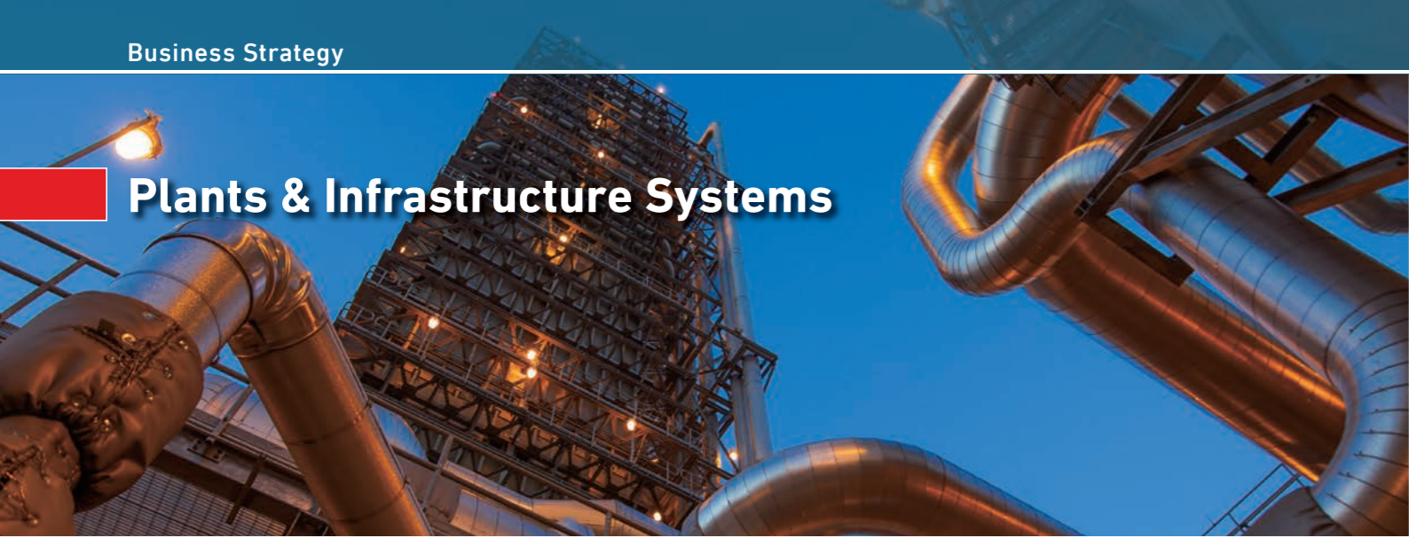
CO 2 Capture Plant (U.S.)
