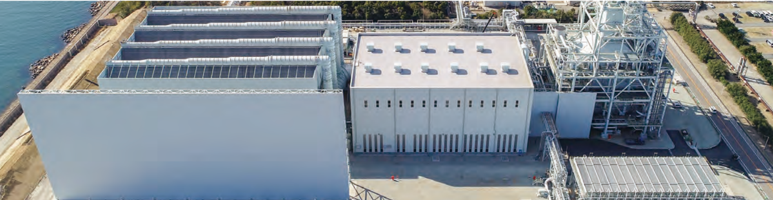
Takasago plant, combined cycle demonstration power plant, No. 2 power generation facility
