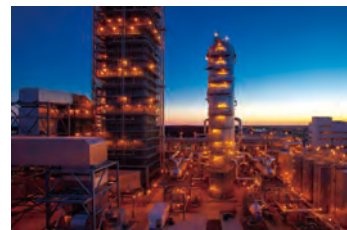
CO 2 capture plant (world's largest CO 2 capture volume of 4,776 tons / day for a power plant application)
