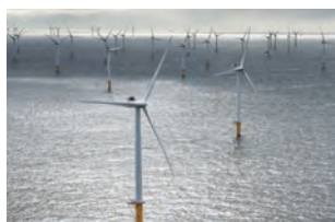
Offshore wind farm
