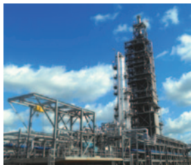
CCS demonstration plant
