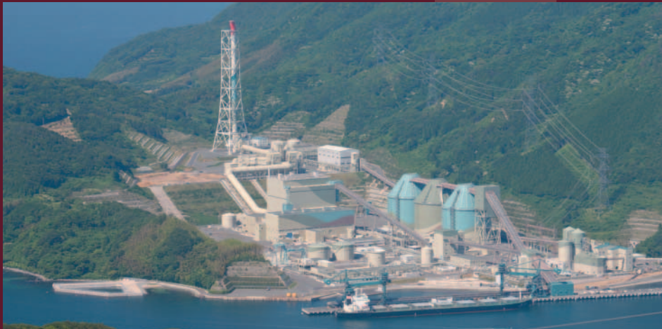
Maizuru No.1 Thermal Power Station of The Kansai Electric Power Co., Inc.
