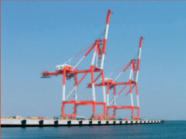
Container Handling Quayside Crane
