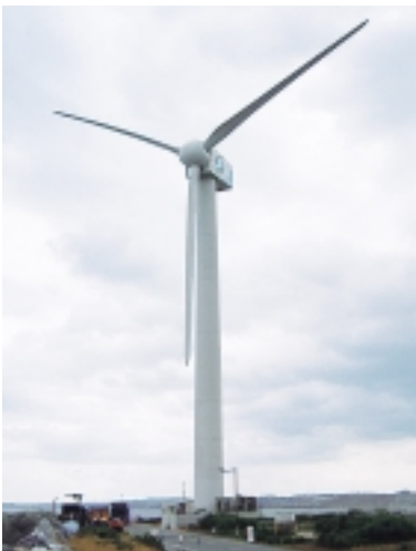
MWT-S2000 Wind Turbine
