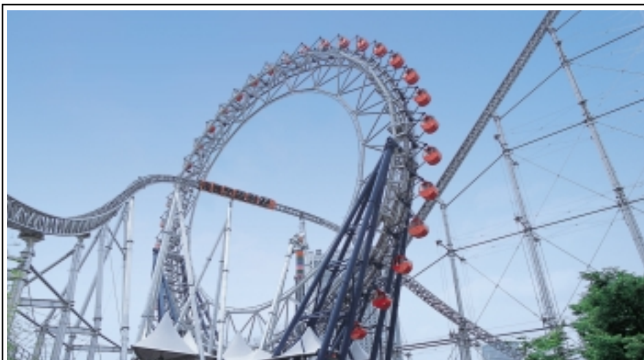
Ferris Wheel "Big O" (Tokyo Dome City) The innovative design of the world's first center-less Ferris wheel allows a roller coaster to run through it.
