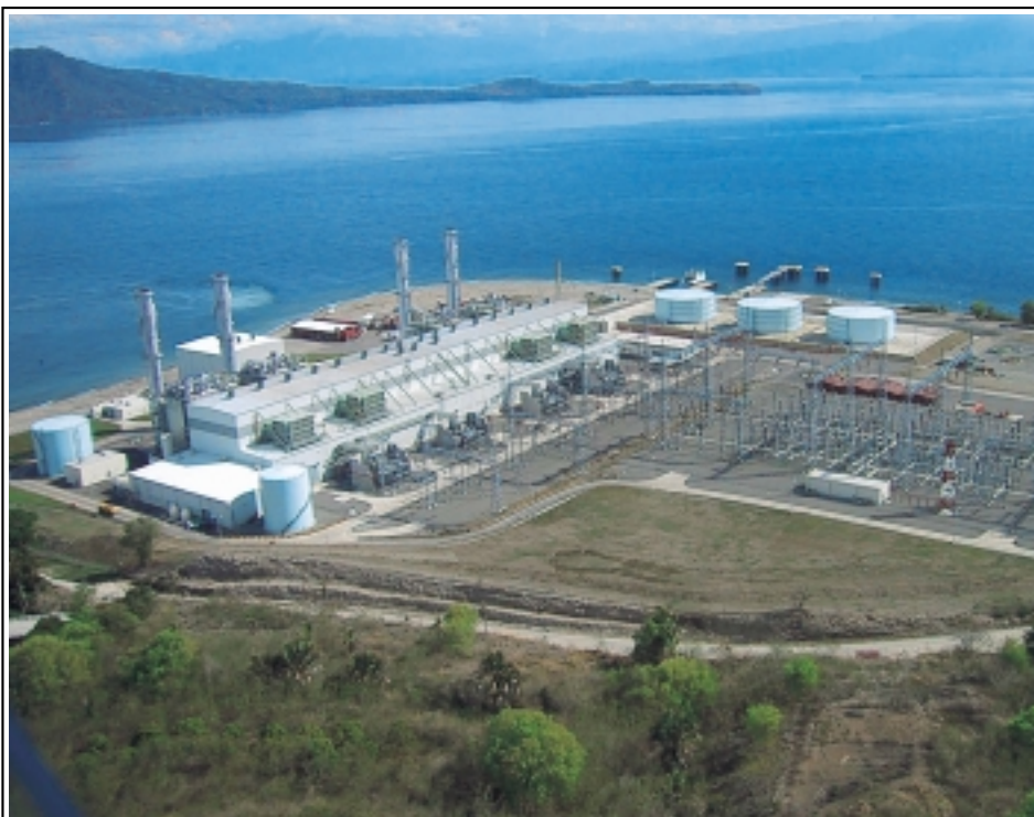
Ilijan Combined Cycle Power Plant (Philippines)
