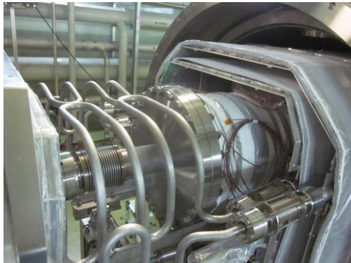
Figure 8: Connection flanges of pipes
