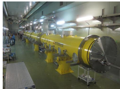
Figure 5: Cryomodule for STF
