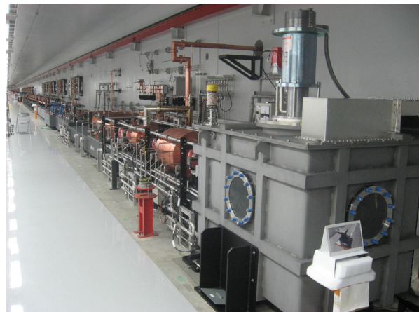
Figure 10: Installation of injector section (by MHI).
