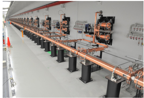
Figure 9: Installation of C-band section (by RIKEN).
