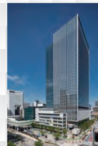
msb Tamachi (港区) [収容台数:110台]
