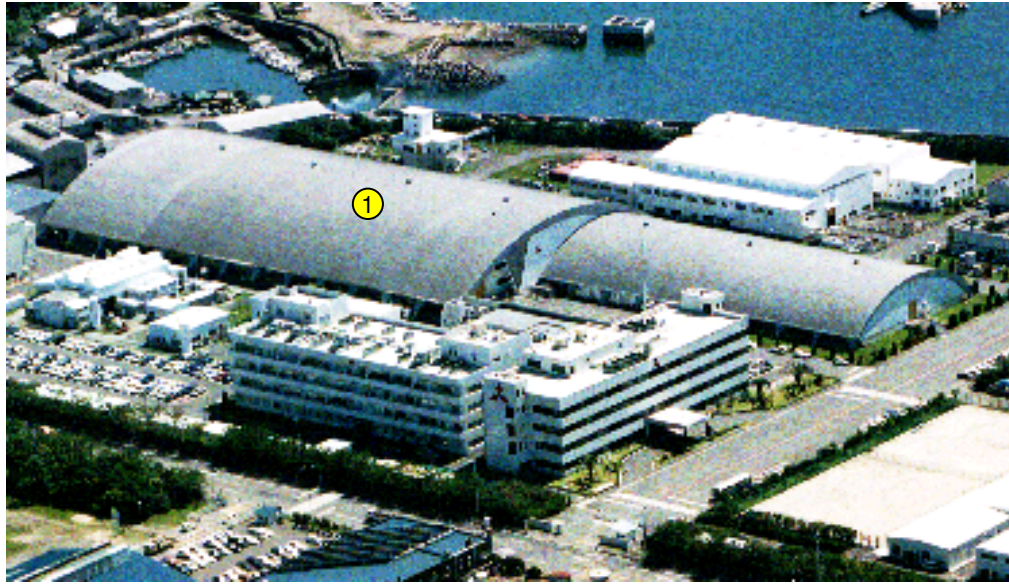
① Seakeeping & maneuvering basin (LxBxD = 160.0 m x 30.0 m x 3.3 m)
