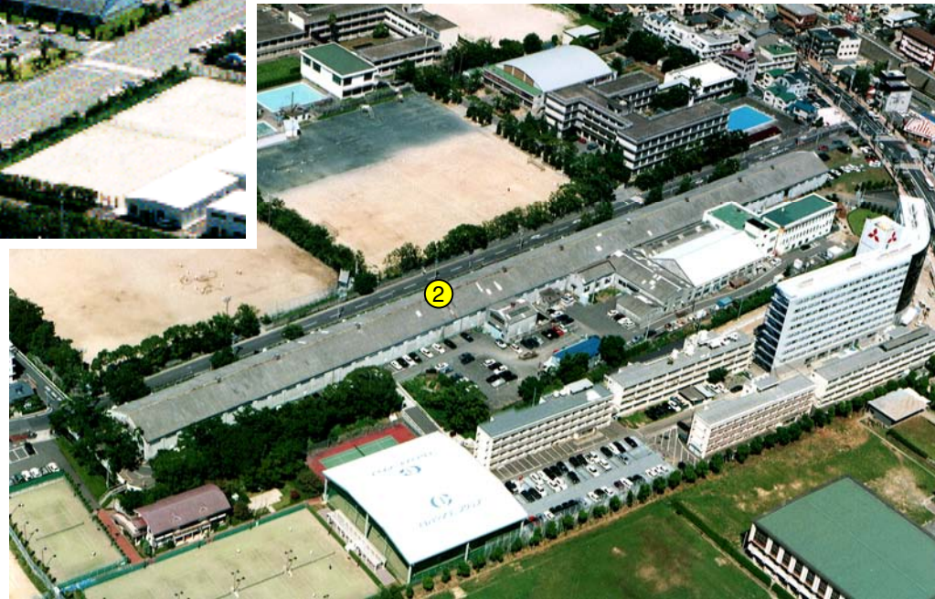
② Towing tank (LxBxD = 285.0 m x 12.5 m x 6.5 m)
