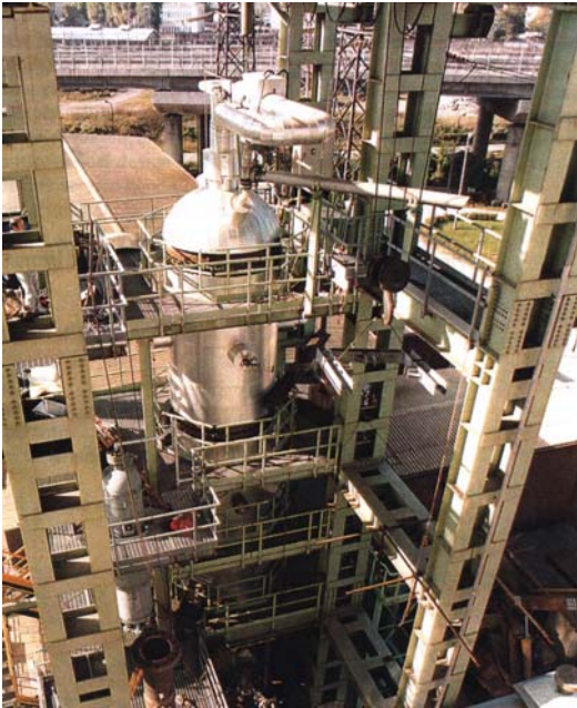
High pressure high temperature tests for steam-water separators of steam generator
