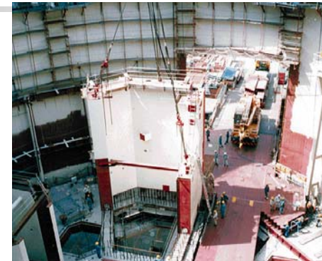
Internal structures using SC (steel plate reinforced concrete)
