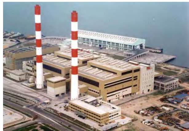
Waste incinerator facility for Singapore
