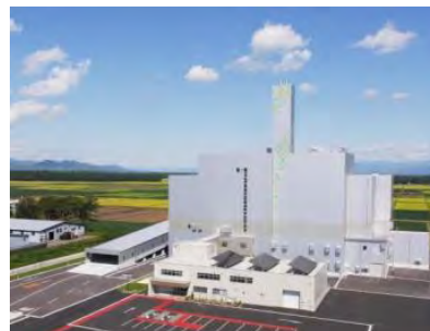
Broad-based association of local municipal offices in central Iwate Prefecture/ Iwate central Clean Center 182t/day(91t/day×2units) Completed Sep. 2015
