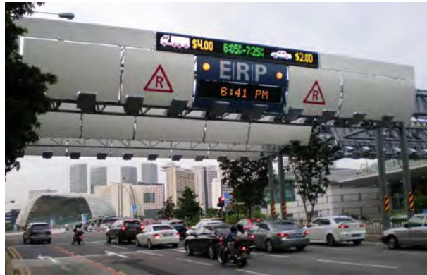
Toll collection system for Singapore
