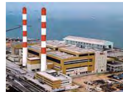
Singapore Government National Environment Agency/TUAS-SOUTH Completed Mar. 2000 4,320t/day (720t/day×6units)
