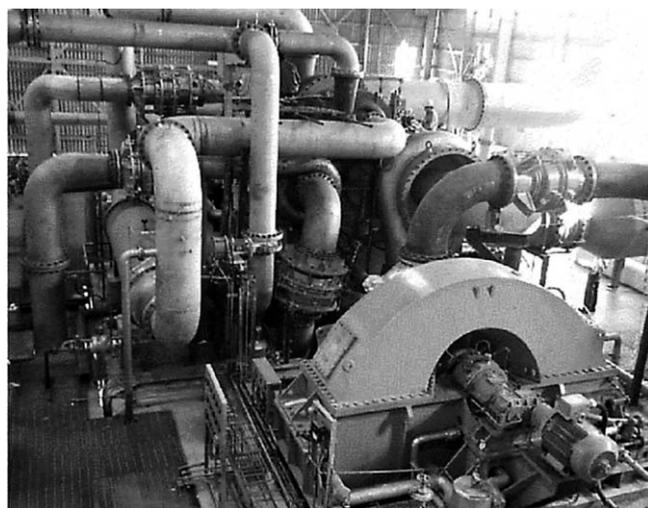
**Fig. 5** Combined geared compressor for PTA plant
