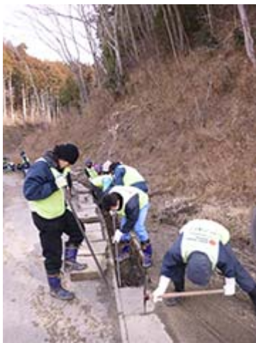
Removing sediment from a drainage ditch
