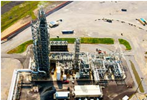
CCS demonstration plant in the U.S.
