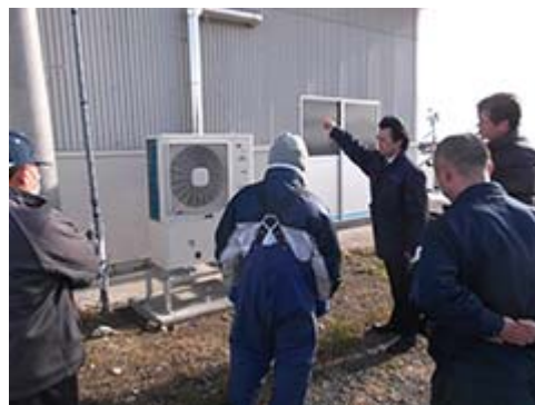
Staff member explains features of the prefab refrigeration unit
