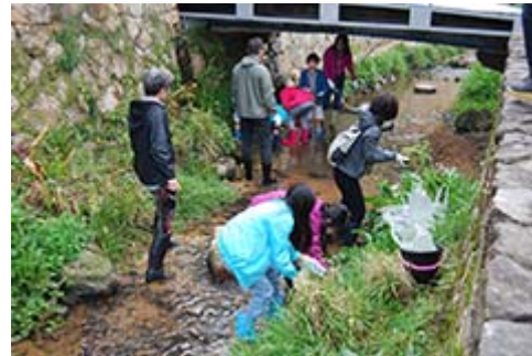
Planting and laying stones in the river
