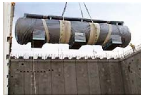
Sludge storage tank installation
