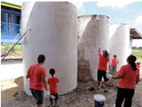
Repairing damaged school buildings
