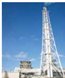
Shin-Sendai Thermal Power Station
