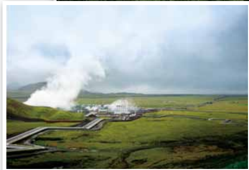
Top: Olkaria II geothermal power plant, Kenya Bottom: Hellisheidi geothermal power plant, Iceland
