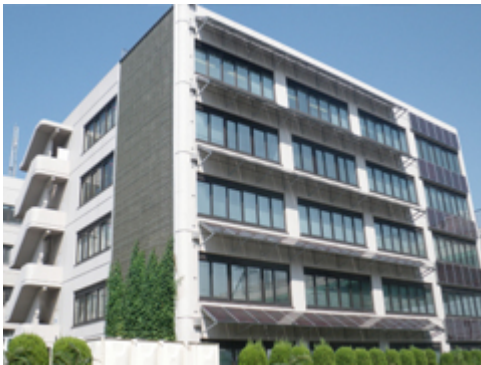
Photovoltaic generation panels installed on the wall of the Ryokoh Building's South Wing
