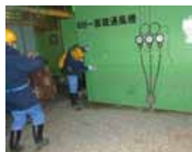
Employees inspecting for damages
