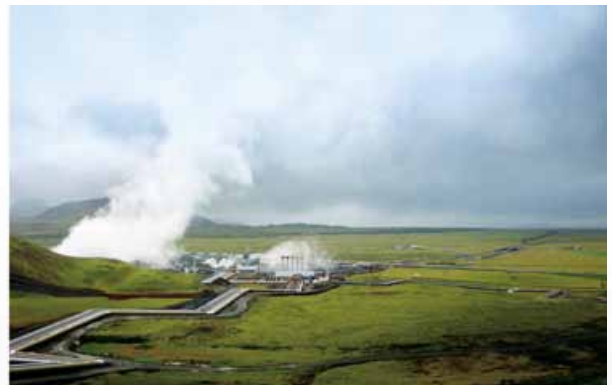
Hellisheidi geothermal power plant (Iceland)
