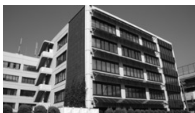
Photovoltaic generation panels installed on the wall of the Ryokoh Building's South Wing
