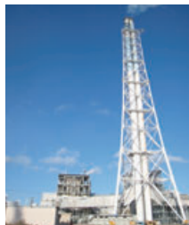
Shin-Sendai Thermal Power Station
