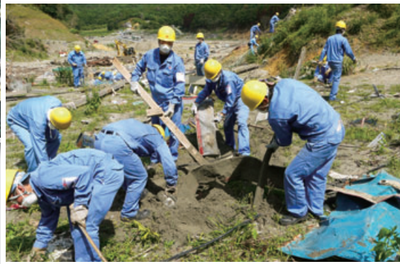
Rubble clearing at a fishing port by Kobe Shipyard & Machinery Works
