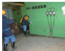
Employees inspecting for damages
