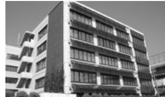
Photovoltaic generation panels installed on the wall of the Ryokoh Building's South Wing
