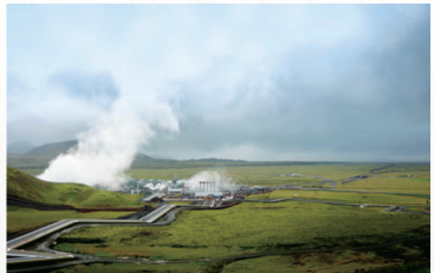
Hellisheidi geothermal power plant (Iceland)
