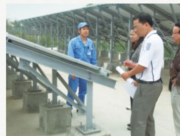
Explaining the use of solar power generation equipment
