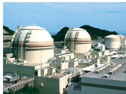
Ohi Nuclear Power Station
