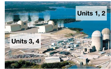
Comanche Peak Power Station of U.S. Luminant Generation Company (Rendering of Units 3 and 4)
