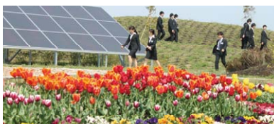
Solar panels installed in the park
