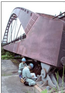
Safety inspection of bridges
