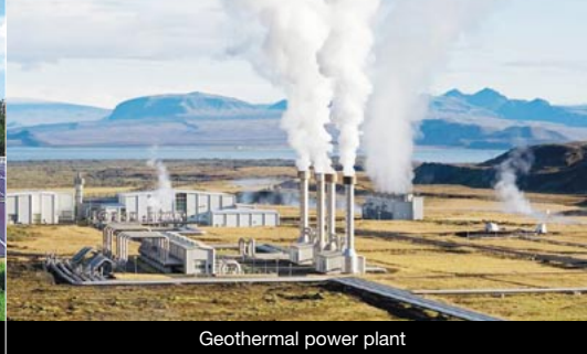
Geothermal power plant
