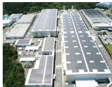
Solar cell panel installed at the microcrystalline-Si tandem-type photovoltaic solar cell second plant of the Nagasaki Shipyard & Machinery Works Isahaya Plant
