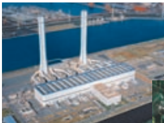
Combined cycle power generation plant
