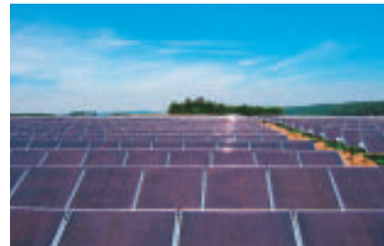
PV plant in Buttenwiesen, Germany 10,000 panels of 100W capacity have been installed.
