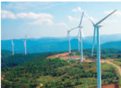
1,000 kW wind turbines at Shikamachi Wind Farm, Nagasaki Prefecture 15 units of 1,000 kW wind turbines have been placed in service for Nagasaki-Shikamachi Wind Power Co., Ltd.
