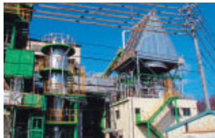
Biomass gasification power generation system for MIE CHUO KAIHATSU Co., Ltd. The system can process 96 tons of wood chips per day to produce 1,400 kW of electricity.
