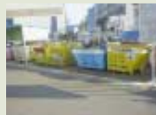
Waste materials separation on carrier ship repairing site
