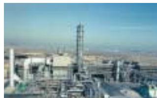
Natural Gas Reforming Plant
