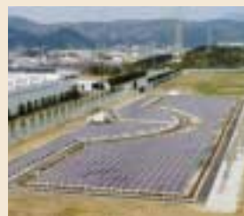
Solar Power-Generation Systems
