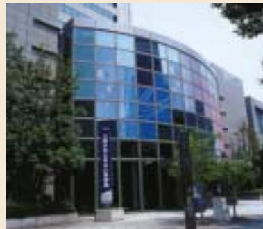
Appearance of Mitsubishi Minato-Mirai Industrial Museum
