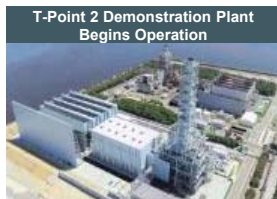
Facility for long-term validation of next-generation high-efficiency JAC* class GTs, which were the first in the world to achieve inlet temperatures of 1,650°C *JAC: J-series Air-Cooled
