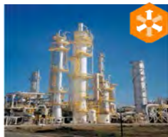
CO2 recovery plant
