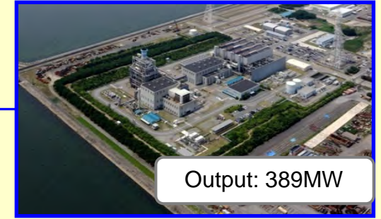
Demonstration facility (Takasago Machinery Works)
