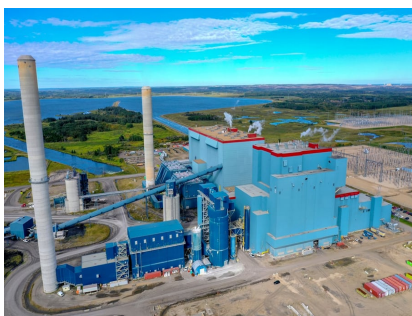
Genesee Generating Station (Alberta, Canada)
