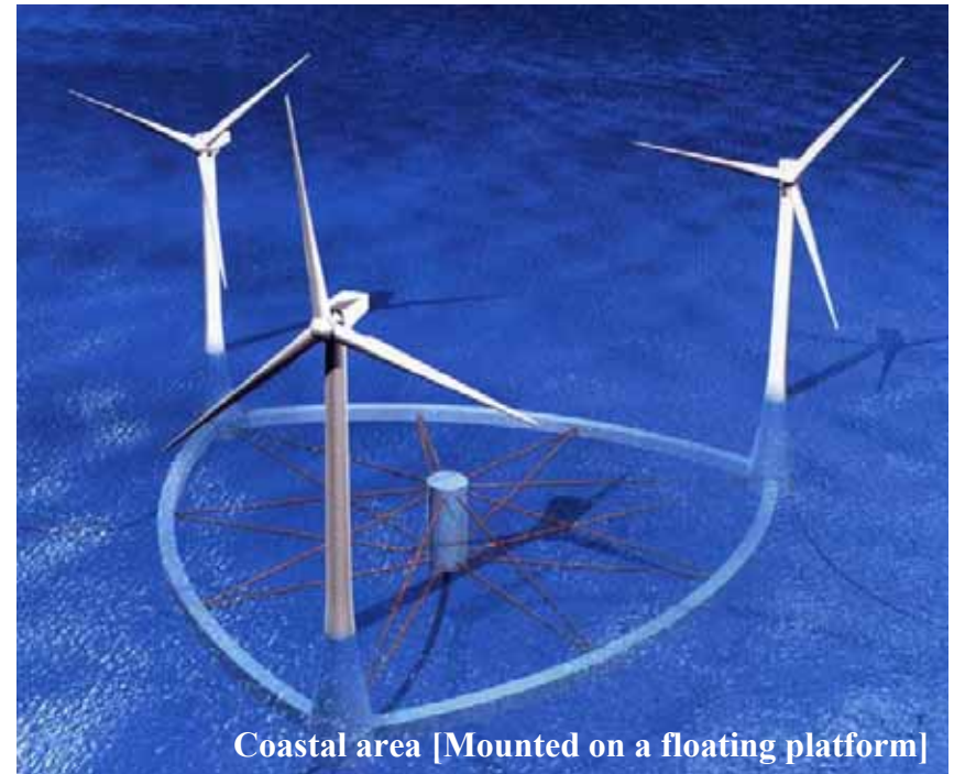
Example of offshore wind turbines mounted on a floating platform (Tokyo University)
