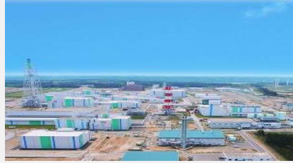
Rokkasho Reprocessing Plant
