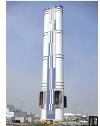
Smokestack for thermal power generation plant
