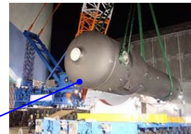
Steam Generator Replacement (SGR)
