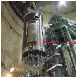
Core Internals Replacement (CIR)
