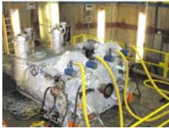
Emergency gas turbine generator
