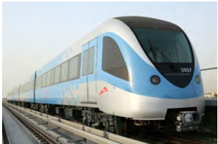
Rail transit system
