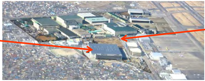
Komaki-minami New Plant panoramic view
