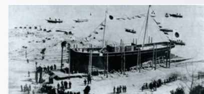
Nagasaki Shipyard & Machinery Works' first steel steamship, the Yugaomaru
