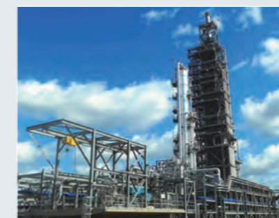
CO 2 capture plant
